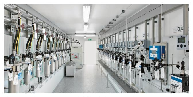
In bigger power plants all quality measurements connected to boiler, boiler feed water and steam condensate are usually centralized monitored in large analytical shelters (Source: Dr. Thiedig GmbH & Co KG, Berlin).
